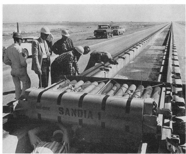
SEVERAL SANDIANS inspect a sled following its run on the six-mile Holloman sled track. The rock-
